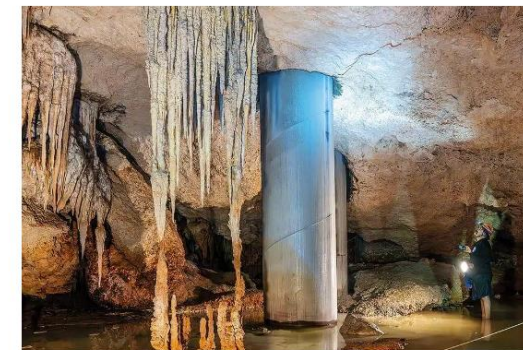
Campaigner Guillermo D Christy stares at one of the giant pillars driven through the karst to support the new train line (Photo: Valentina Cucchiara)
